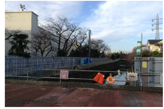
かなな橋を望む (上流側) (View of Kanna Bridge from the upstream side)
